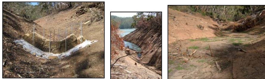
Figure 4 (Above) Hay bale traps pre, during and post reservoir water level rise. Figure 5 (LH Below) Traps needed to be larger than the creek channel
