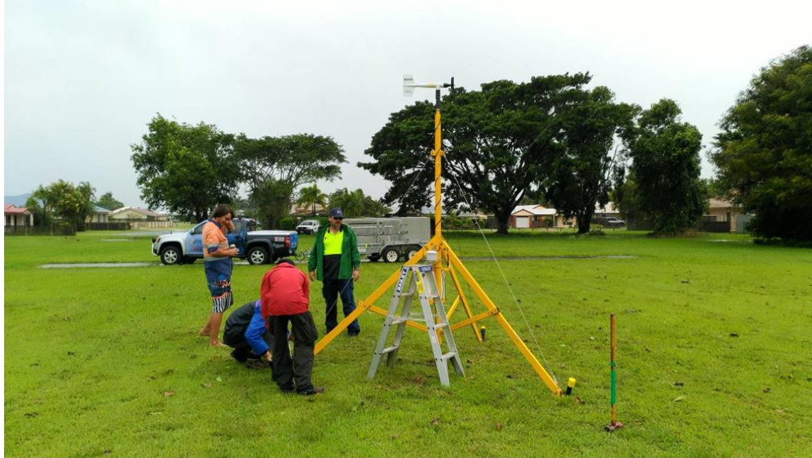
(a) Tower installed before cyclone
