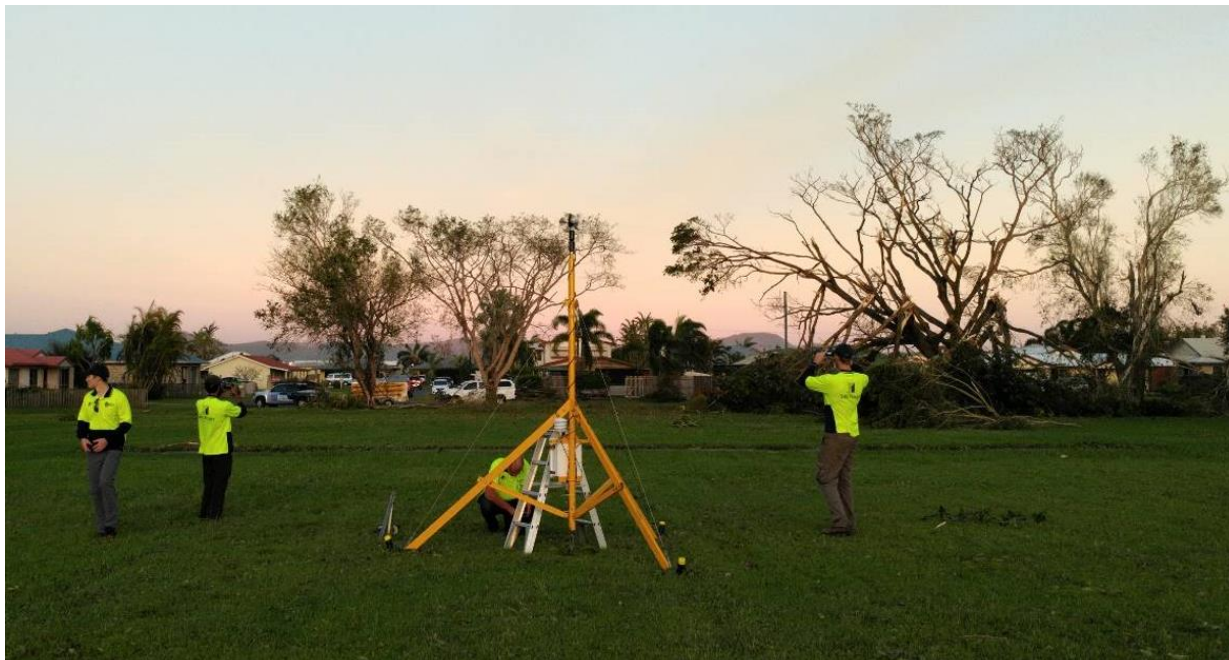
(b) Dismantling tower after cyclone
