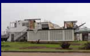
Damage to pre-Tracy home (Cyclone Yasi, Cardwell)
