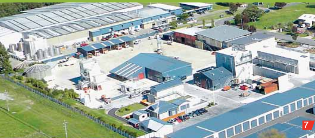
7: The entire site is environmentally friendly, using a firefighting water supply that is pumped through the fire mains to be used for training. The water is then captured in a retention pond, treated and reused. All live burn training is conducted indoors and the smoke is treated through a thermal oxidiser to comply with requirements of the nil smoke emission resource consent that is in place for the site. The scenarios consume many resources and take considerable time to prepare. Nowadays the obvious environmental effects of water runoff and smoke are becoming very difficult to defend.
